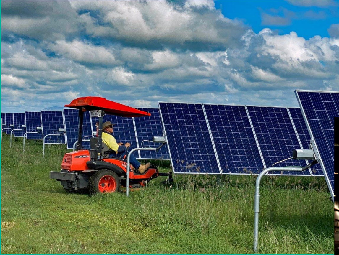
Queensland solar farm.
