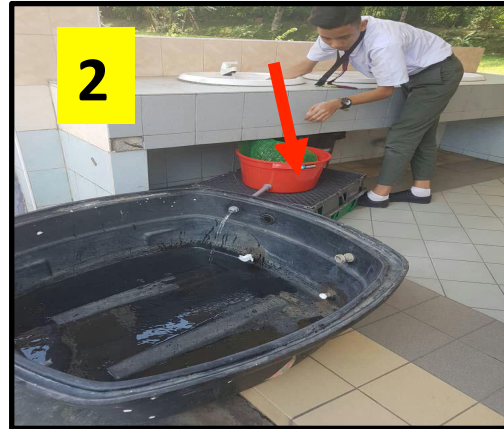
Place the filter under the sink
